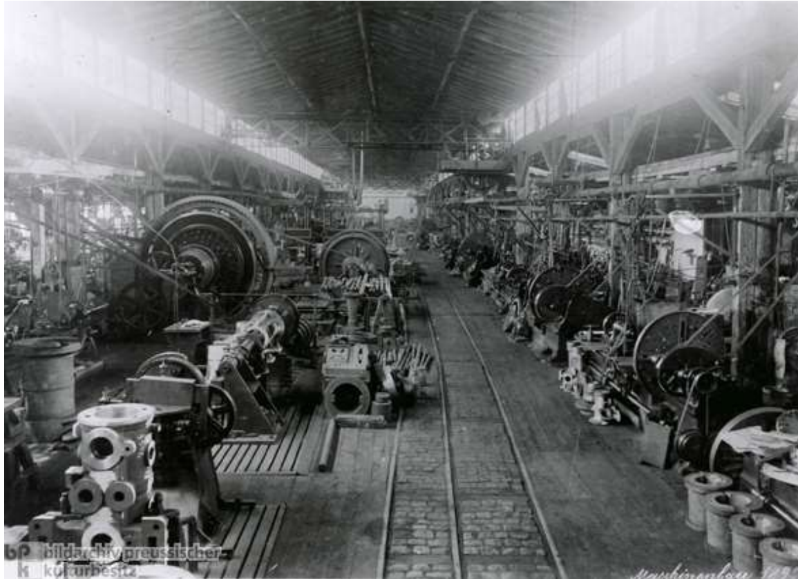
Machines driven by belts from an overhead lineshaft
